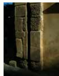
Groove for the portcullis in the central opening.
