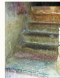
Stairs at the side entrance.
